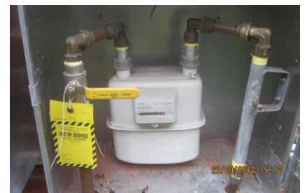
Fabricated meter bend examples
