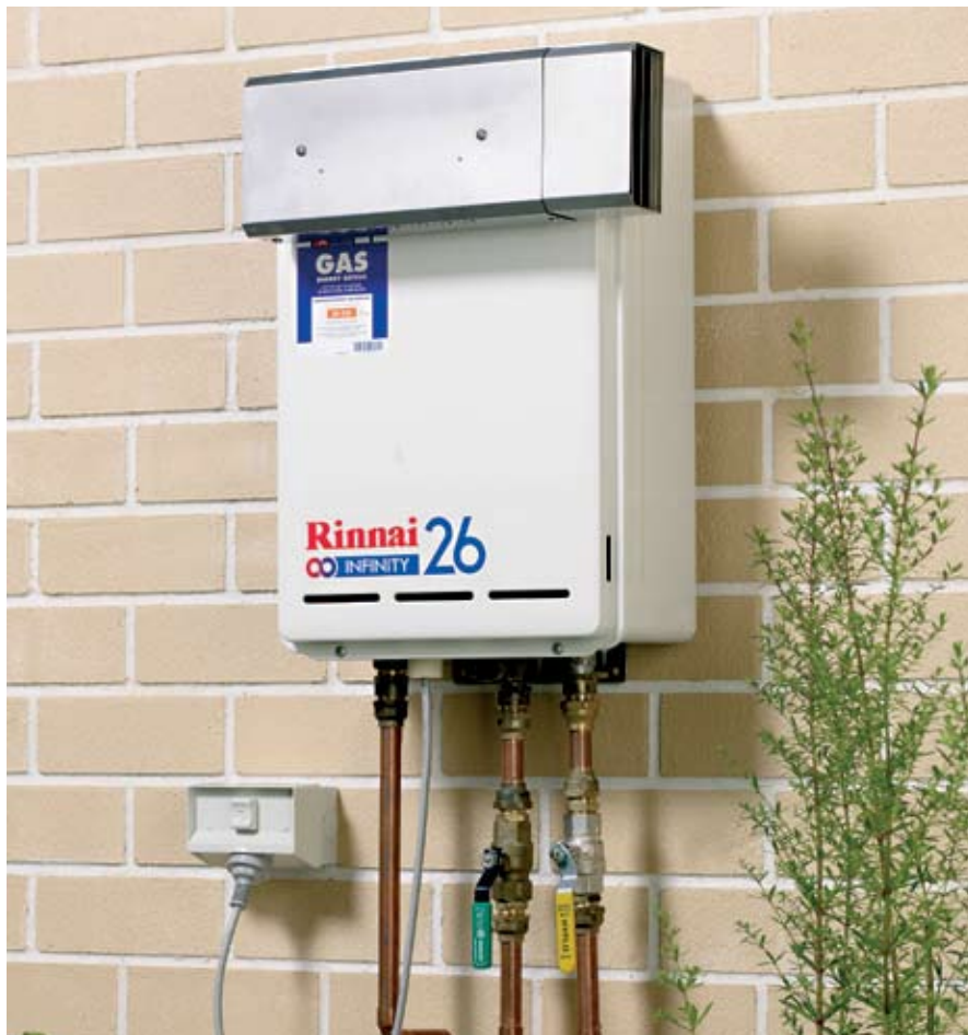
Side flued water heater suitable for installation in a covered area with only one side open
